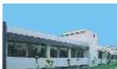
Roto's Manufacturing Plant
